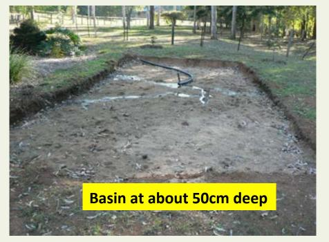
The easiest and cheapest way is to plant directly to the ground into a basin, which is needed to prevent effluent runoff to surrounding area. However this method may incur deep drainage, which is not allowed by EPA on some soil types
